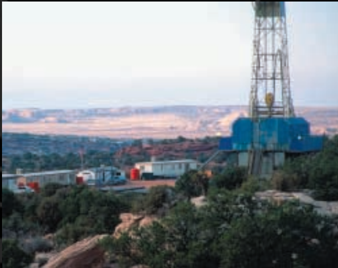
Conoco well in the Grand Staircase Escalante National Monument © John Palmeri
