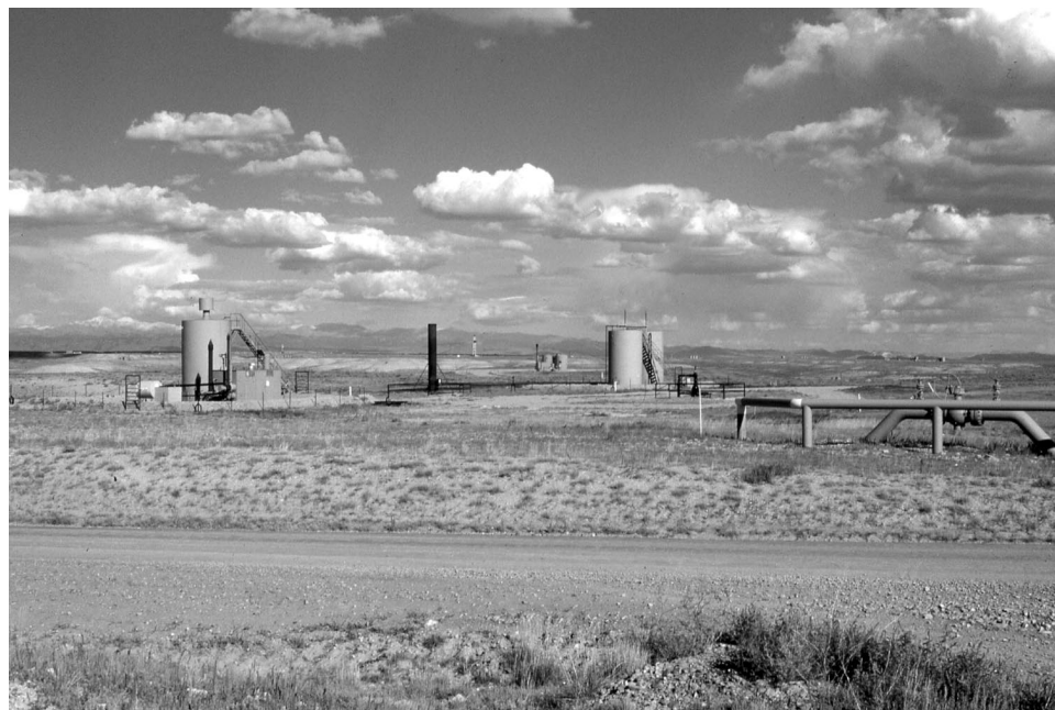
Figure 3: Typical Oil and Gas Site Subject to an Environmental Inspection
